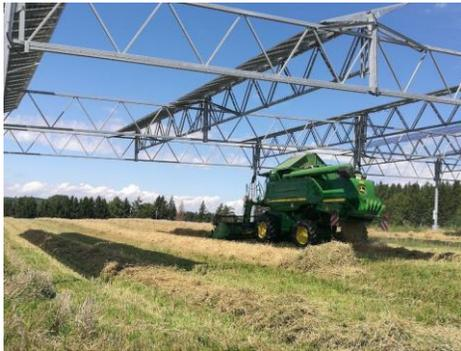
**Agrophotovoltaics** being tested in Vietnam and Chile use solar panels on stilts above cropland to gather energy while growing crops. Panels produce shade and make enough electricity to cool, clean and package the produce.
