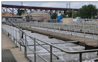
Aeration tanks at the Wards Island plant
