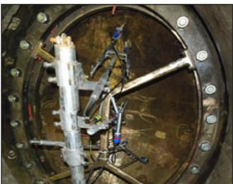
**Now:** Today, the bronze access door is a key element in ongoing work to repair the Delaware Aqueduct. In order to ensure that the tunnel can be dewatered safely, extensive research is being done by DEP engineers and contractors on the structural history and installation of the bronze access door. (Photograph by Ted Dowey; 1/23/2010)
